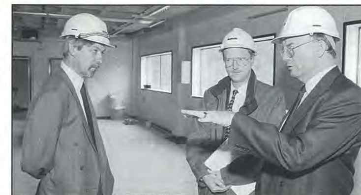
Duncan Whyte is pictured inspecting building work underway at the Caernarfon Depot with Network Manager Colin Blundell, left, and Building Engineer Selwyn Jones.
